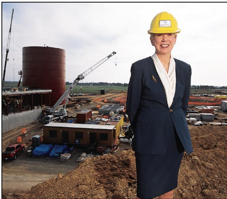
The first buildings are rising at UC Merced, where Carol Tomlinson-Keasey has been chancellor since 1999.
